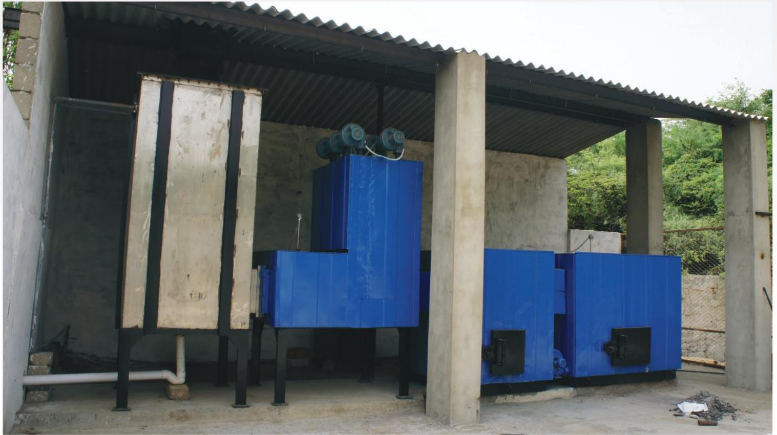
The GT50 with cooling chamber and SS Wet Scrubber. Made for the Combined Military Hospital (CMH) Malir Cannt.
